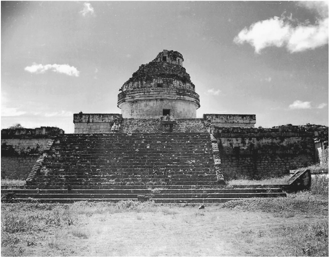
Fig. 9.5. The Mayan “observatory” at Chichén Itzá. From the observing platform of the Caracol ancient Mayan astronomers had a clear line of sight above the treetops. The various windows in the structure align with the risings and the settings of Venus and other heavenly bodies along the horizon.
